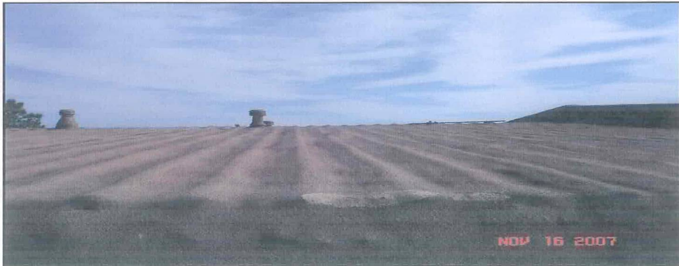
39. This photograph shows another view. These problems with the blistering and irregularity are general problems throughout, yet the patches never addressed these problems.
