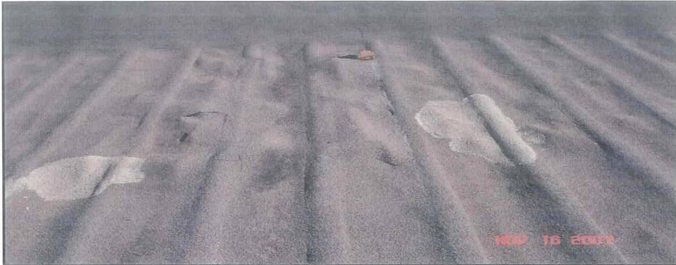
39. This photograph shows another view. These problems with the blistering and irregularity are general problems throughout, yet the patches never addressed these problems.
